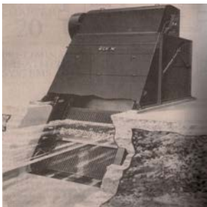
Fig.3: Mechanically cleaned bar screen Source: (Courtesy Envirex, a Rexnord Company.) Cited in McGhee, Water Supply and Sewerage, 1991
